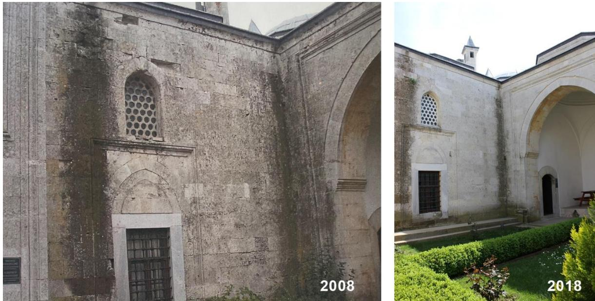
Figure 6 - Before (2008) and after (2018) facade cleaning.
