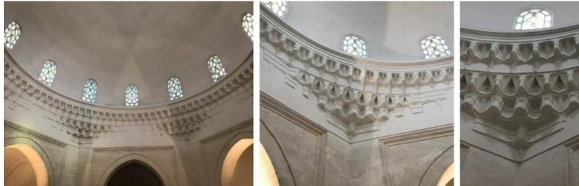
**Figure 18 - Muqarnas used in spaces with their acoustic properties.**
