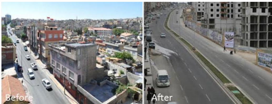
Figure 12 Özdemir Bey Street before and after Urban Transformation project
