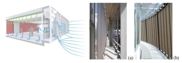
Figure 1. Double skin facade applications, (a) Manitoba Hydro Place [13]; (b) Angel Sguare [16]
