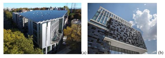
**Figure 3.** Use of photovoltaic panels on the roof and facade, (a) Bullitt Center [17]; (b) Bursagaz Administration Building [21]
