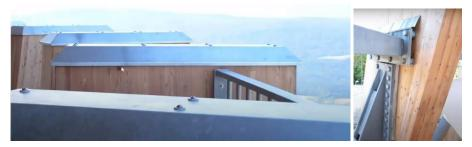
Figure 1. a; metal caps for columns, b; dropper detail (Aklan, 2021)
