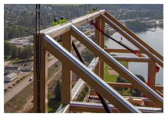
Figure 2. Metal caps for the top frame (CTBUH, 2021) (Photo: Moelven)
