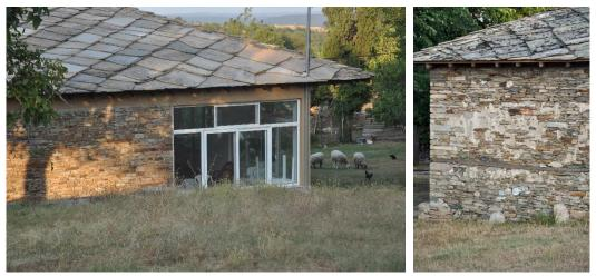
Figure 5. Slate stone is used on walls and roof
