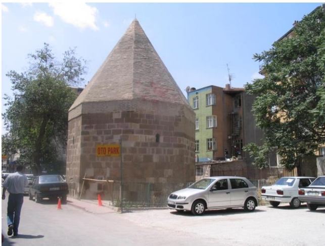
Figure 4. The historic building wall surface made by stone and brick material and belonging to Seljuk Empire
