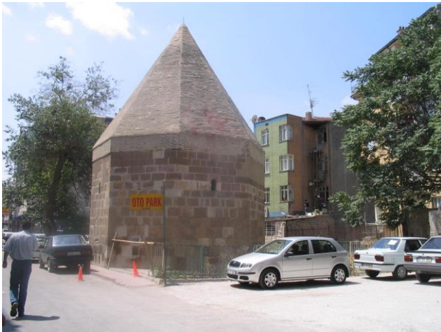
Figure 4. The historic building wall surface made by stone and brick material and belonging to Seljuk Empire
